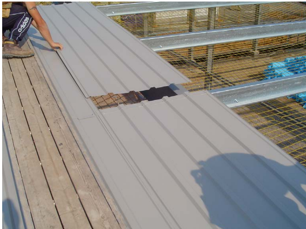
Figure 2.4 Liner sheet installation progressing into the span of the purlins.
