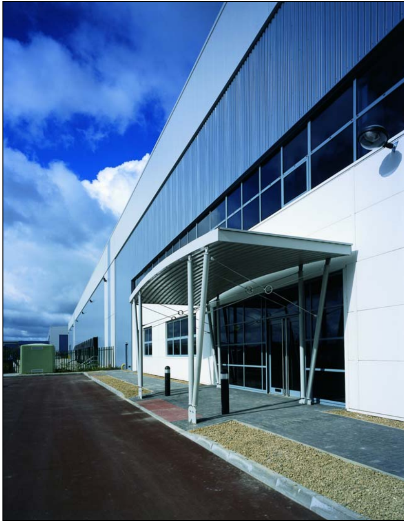
Figure 3.1 Typical wall cladding with a mix of flat panels and profiled sheeting
