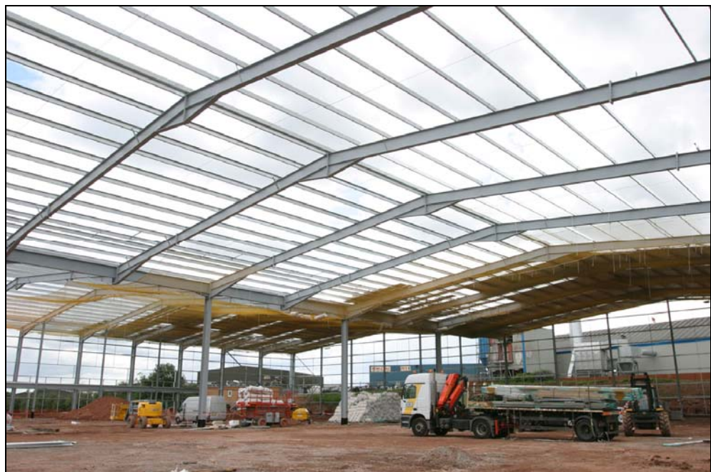
Figure 4.1 Purlins spanning between rafters in the roof
